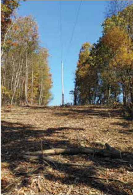
EASIER ACCESS: A recently trimmed and maintained right of way near Taylor Hill Road in Glen Rock will allow for easier access for crews when an outage occurs.
